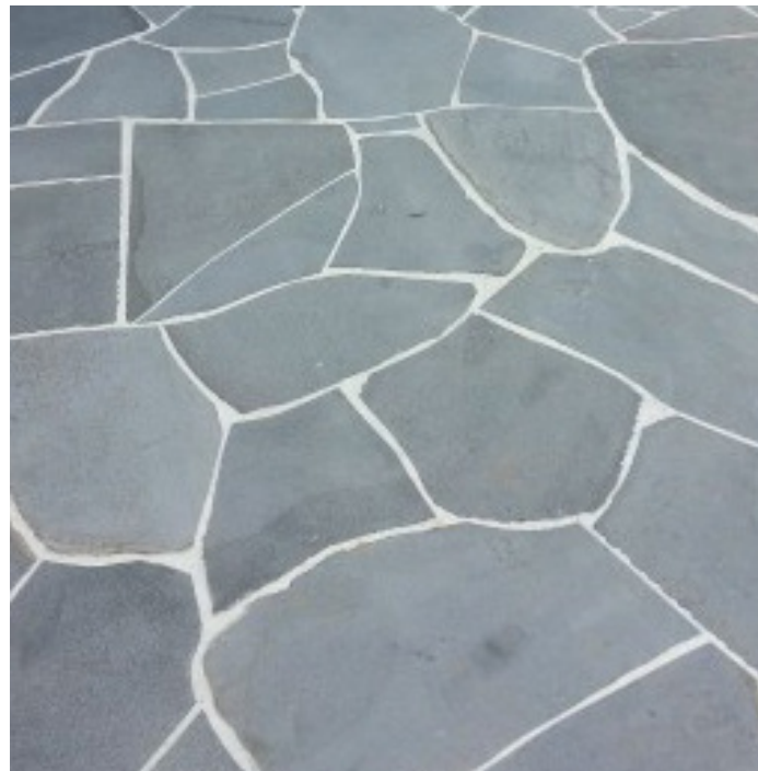
Paving Type 4. Product: Yorkstone slabs, irregular shapes with 'green' joints Supplier: Marshalls or Similar Approved Size/Colour: max. 800x800x80mm
