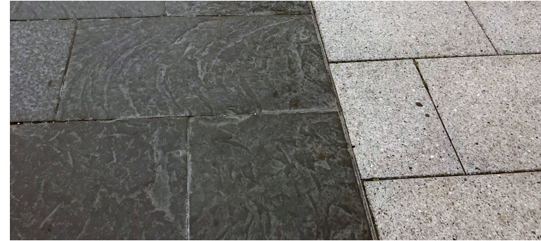
Paving Type 2. Product: Granite slabs Supplier: Marshalls or Similar Approved Size/Colour: 300x450x80mm/Dark grey
