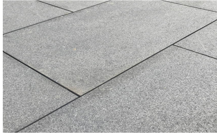
Paving Type 1. Product: Granite slabs Supplier: Marshalls or Similar Approved Size/Colour: 700x450x80mm/Light grey (Silver grey)
