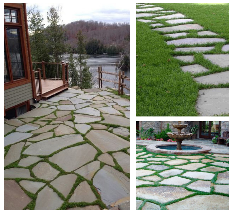
Paving Type 5. Product: Natural stone slabs, irregular shapes with 'green' joints Supplier: Marshalls or Similar Approved Size/Colour: max. 800x800x80mm
