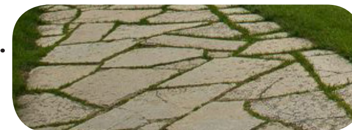
Semi-hard path along the hard surfaces with mortar joint. The 60-80 mm wide grass joints soften up the hard landscape.
