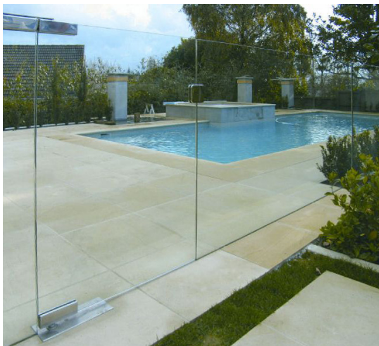
Furniture Type 11.: Frameless Glass Balustrade Supplier: TBC Height: 1.1m
