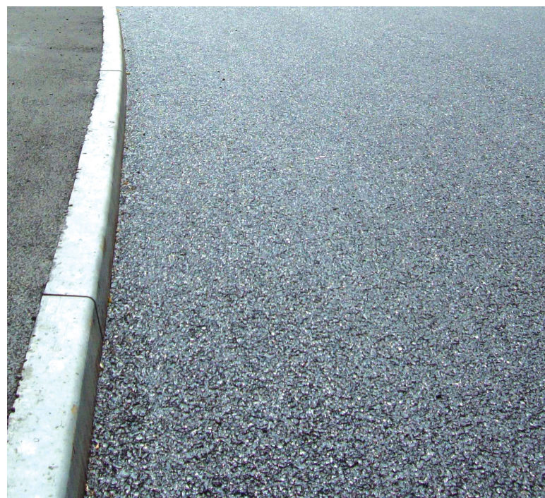
Edge Type 1. Product: Conservation Kerb Supplier: Marshalls or Similar Approved Size/Colour: 145x255x915mm/Concrete/Textured.
