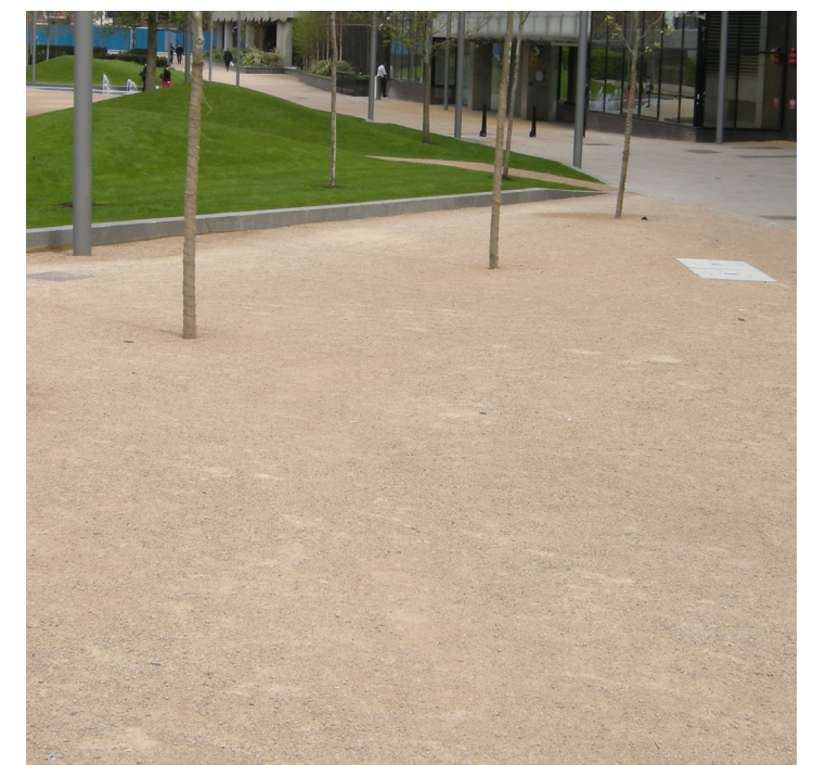
Paving Type 6. Product: Self binding gravel Supplier: Breedon Special Aggregates or similar app. Size/Colour: 0-4mm/ Golden Amber
