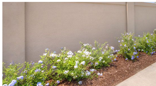
Block work wall with rendered finish. Finish by architects.
