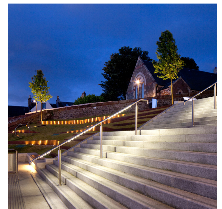
Furniture Type 10.: Handrail Supplier: LiniLED Description: Stainless steel handrail with LED lighting compliant with building regulations.
