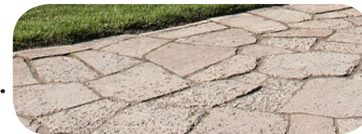
Designated disabled access path - min. 1.5m wide path with 2m long by 1.8m wide passing places on every 25m distance. Paving made with mortar joints rather than green joints.
