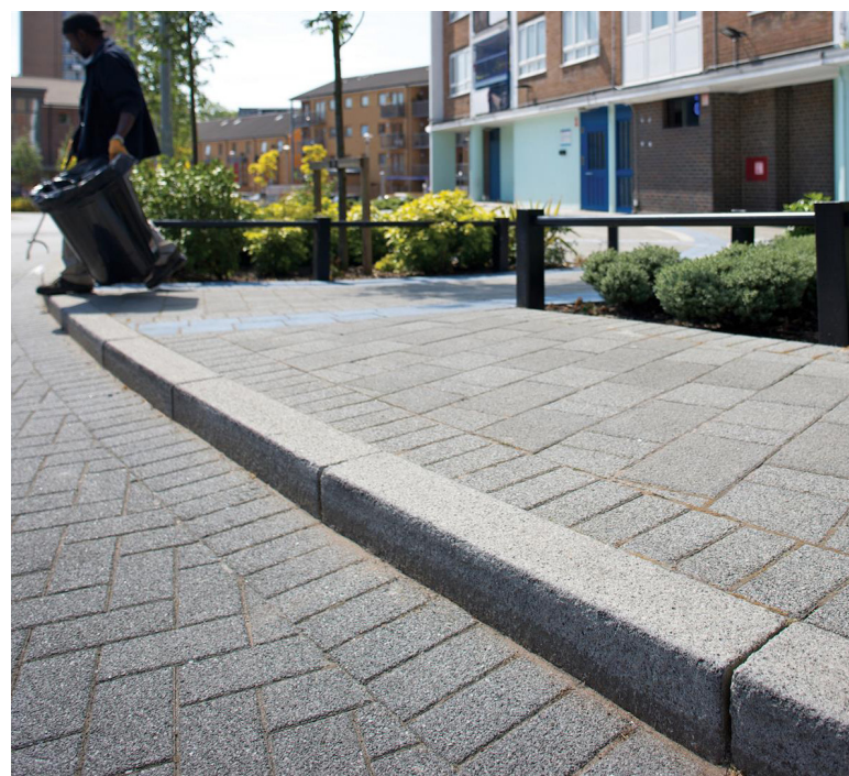
Edge Type 1. Product: Conservation Kerb Supplier: Marshalls or Similar Approved Size/Colour: 145x255x915mm/Concrete/Textured.
