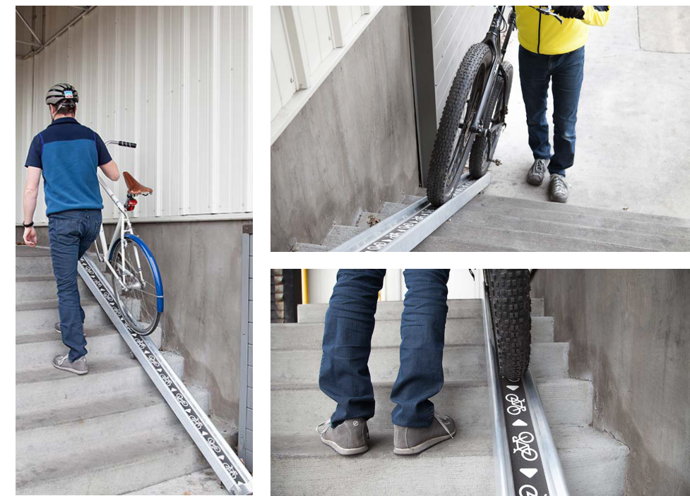
Furniture Type 14. Metal bicycle access channel. (To help move the bikes up and down on the steps.) Supplier: TBC
